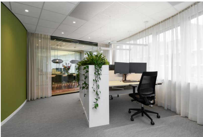
In the office-area SPOT DK is the basic Lighting and LINEAR INDIVILED D/I for the working areas. All luminaires in DALI versions were used in a KNX system.
