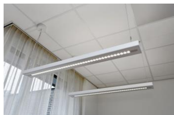
In the office-area SPOT DK is the basic Lighting and LINEAR INDIVILED D/I for the working areas. All luminaires in DALI versions were used in a KNX system.
