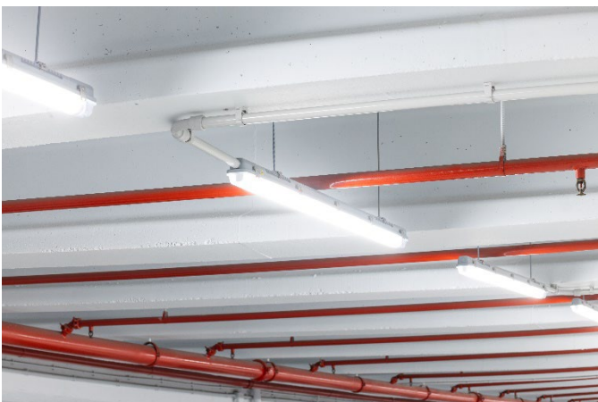
DALI compatible LED T8 tubes allow for more efficient control and monitoring
