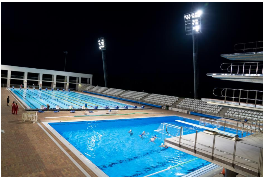
Outdoor pool lighting
