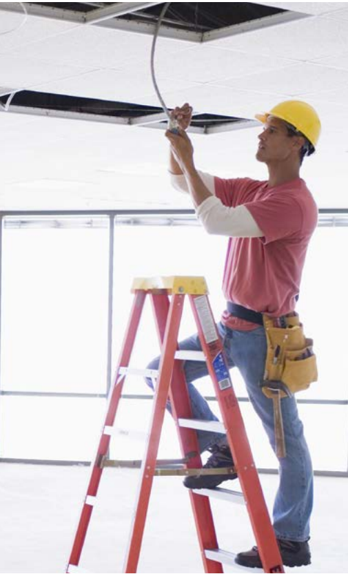
1 Disconnect luminaire from mains
