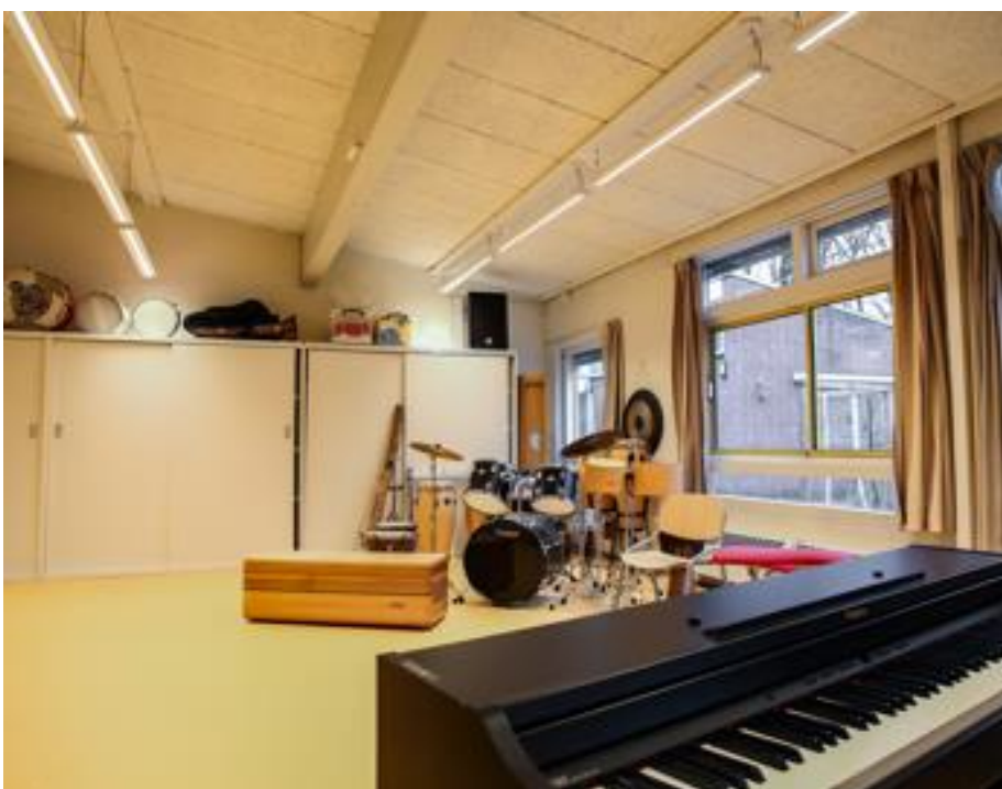
LEDVANCE LINEAR INDIVILED DIRECT DALI luminaires for the classrooms ensure a high quality and glare-free lighting.
