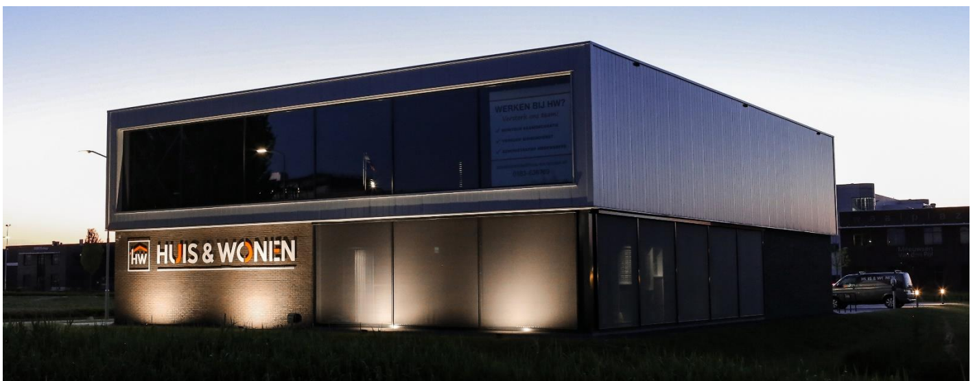
LEDVANCE FLOODLIGHT luminaires ensure an evenly well lit facade and logo.
